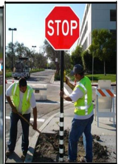
Fig 6.5 traffic sign replacement
